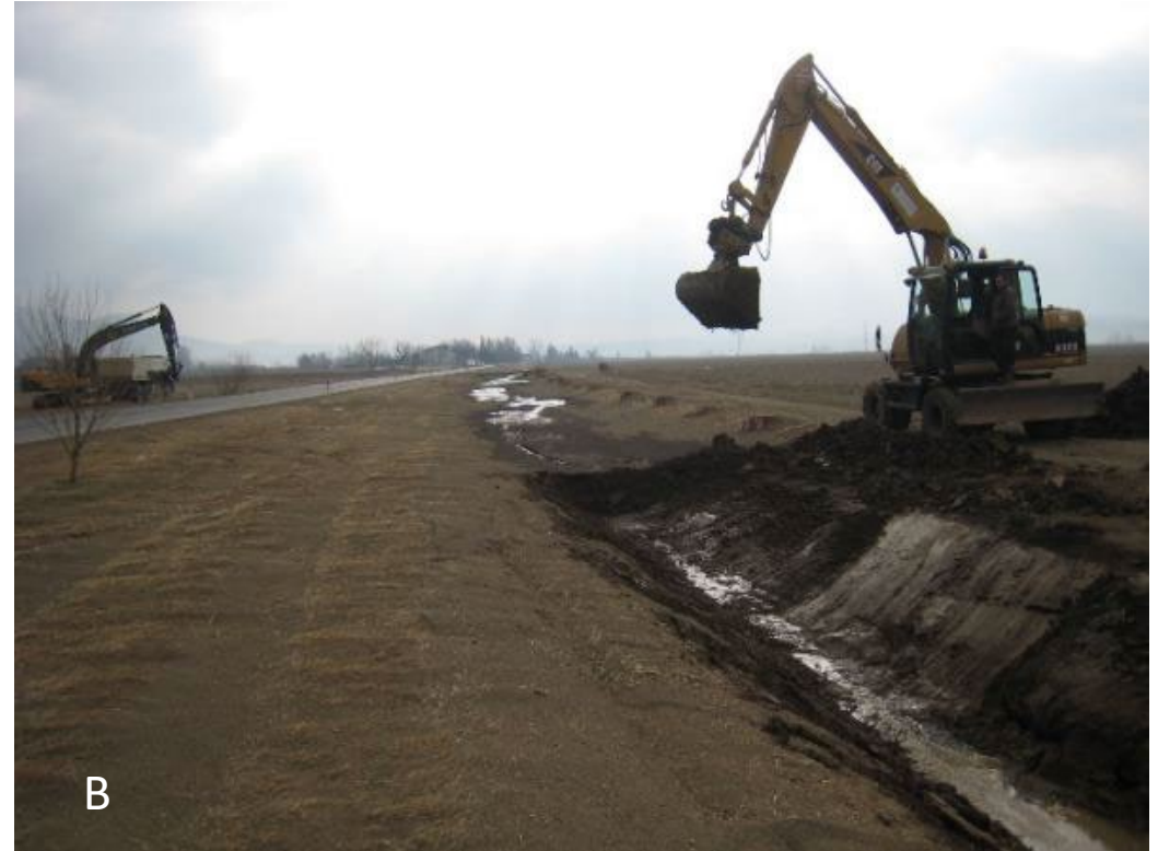
Figure 2: Soil erosion by Bora wind in 2012: (a) drainage ditches levelled with farmland, as they have been completely filled with eroded topsoil; (b) transport of the eroded soil back to the neighboring agricultural land (credits: Uroš Štibilj).
